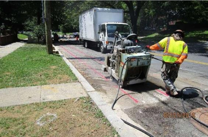
Marked & saw cut
