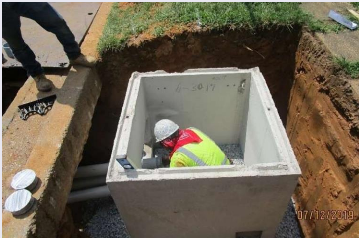
Structure tied into conduit
