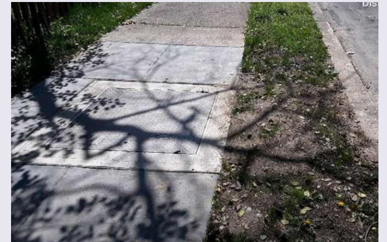
Final restoration tap hole
