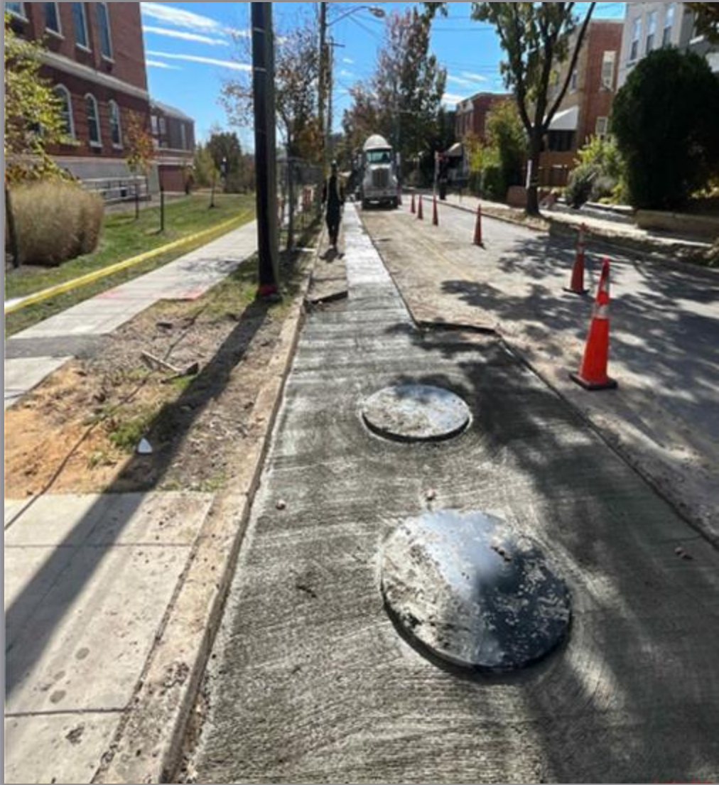
Restoration of manhole
