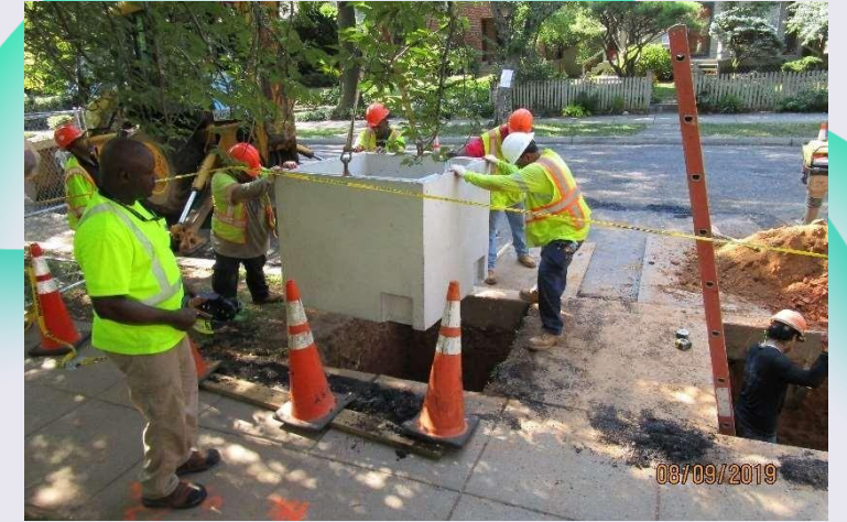
Structures lifted into excavated hole
