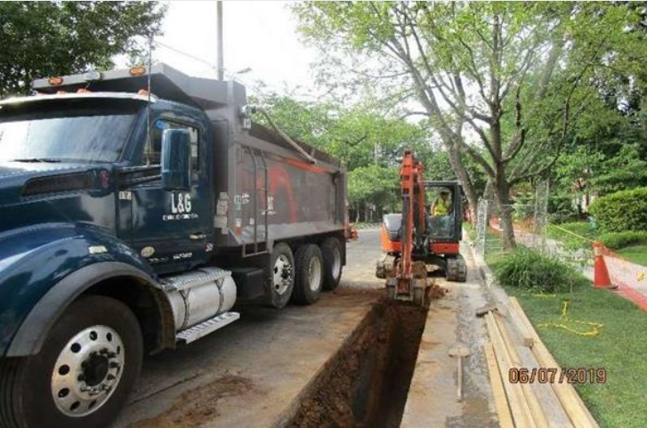
Trench is excavated
