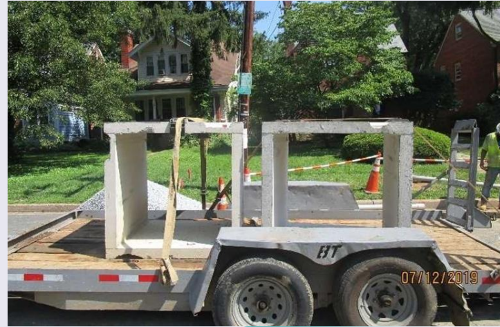
Structures delivered to site
