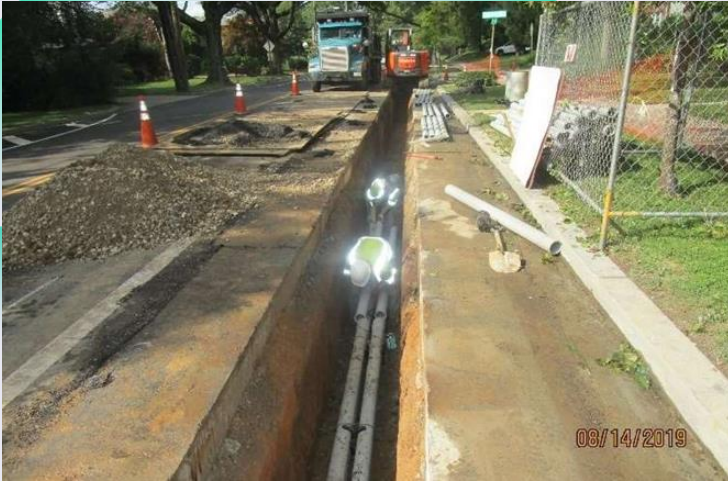
Conduit is laid
