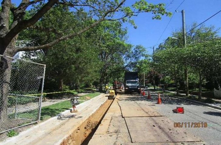
Trench is backfilled, then temporarily covered
