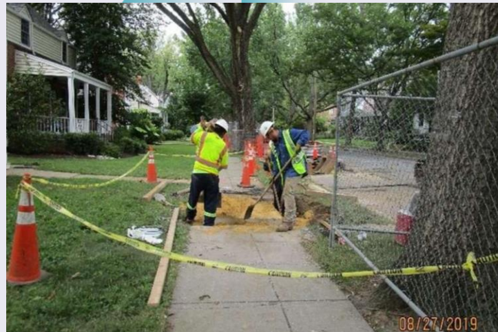
Structure is capped off & backfilled
