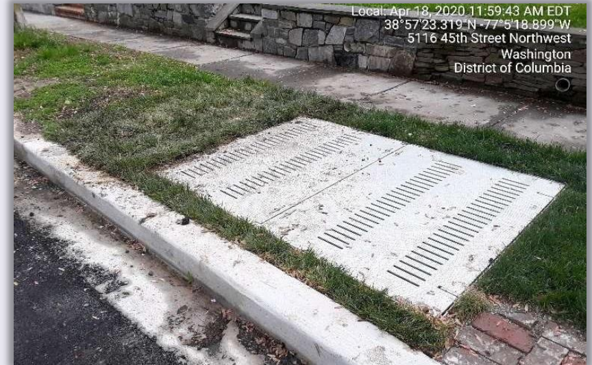
Restoration of transformer enclosure
